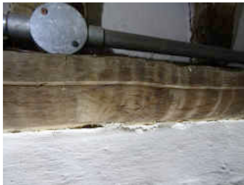
Figure 79 ~ Details showing staining from past leaks.
