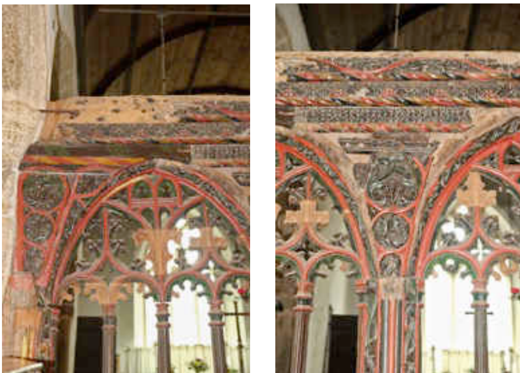
Figure 48 ~ Details showing the bright over paint covering several areas of the architectural framework.
