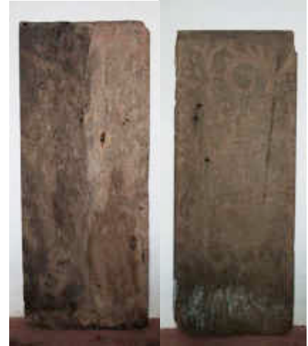
Figure 55 ~ Four panels currently stored in the vestry (above left) and the reverse of the far right two (right) showing rotten decay, dark staining and mould from damp and insect damage.
