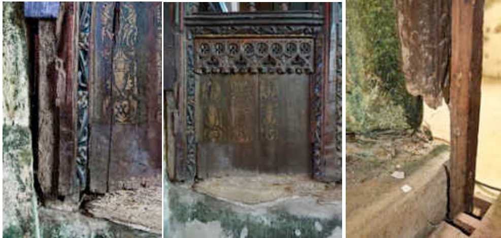
Figure 36 ~ Details showing various areas of losses and vulnerable sections observed across the rood screen.
