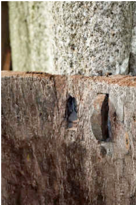
Figure 75 ~ Detail of ferrous fixing, anchoring the upper edge of the pulpit to the adjacent stonework.
