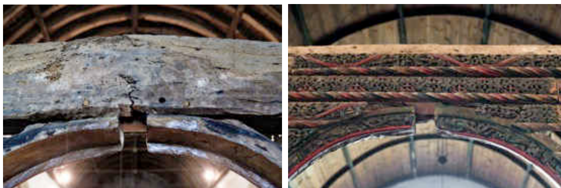
Figure 47 ~ Sections of carvings have been repositioned within the flattened spandrels (top left & right) and run of moulding are misaligned with inconsistent gaps (below left & right).
