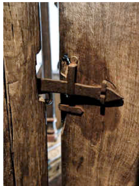
Figure 65 ~ Candle wax drips around attached timber blocks found either side of the book stand (left) and darkened timber adjacent to the door latch and along the top edge of the pulpit from frequent handling and cleaning.
