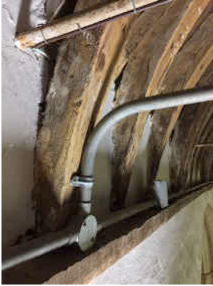
Figure 95 ~ Tie rods were introduced across all three areas of roof timbers during an earlier Victorian phase of repair.
