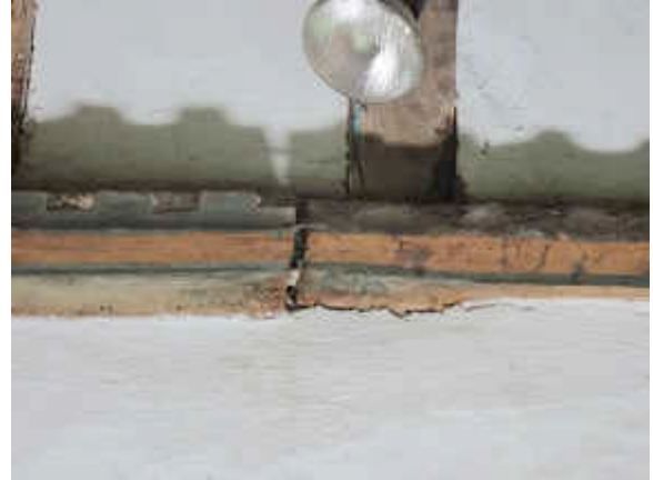
Figure 84 ~ losses to the timber structure in general and to the wall plate line (above right) were observed throughout the church.
