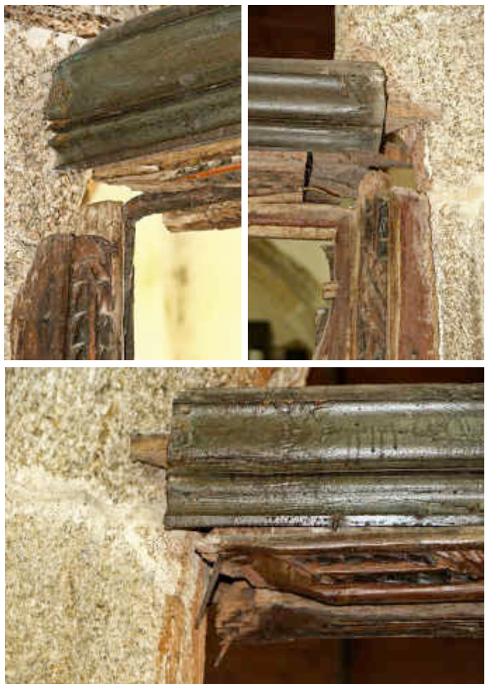
Figure 59 ~ Details showing fixings and ferrous nails through the timberwork. The fixing mechanism to the granite is inadequate.
