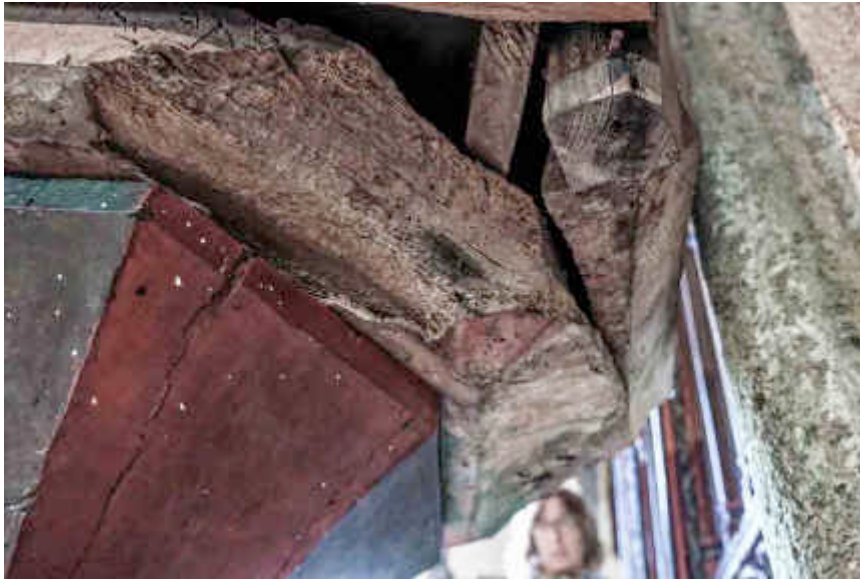
Figure 68 ~ Area of timber at base of pulpit floor (right side of opening) above pedestal showing particularly bad signs of previous insect infestation.
