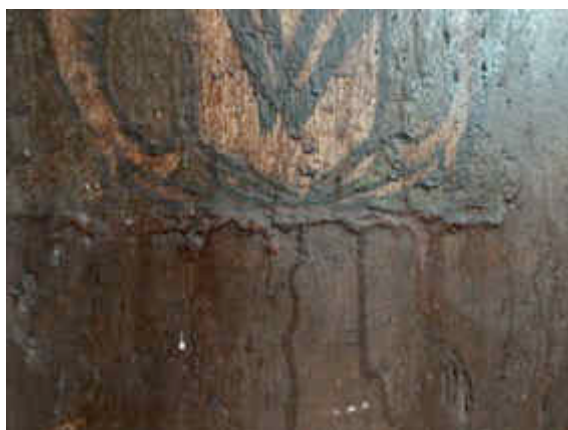
Figure 44 ~ The panels on the west elevation of the north aisle sections of the screen have been coated with a varnish. As noted elsewhere this coating has been thickly applied with dark drip runs observed.
