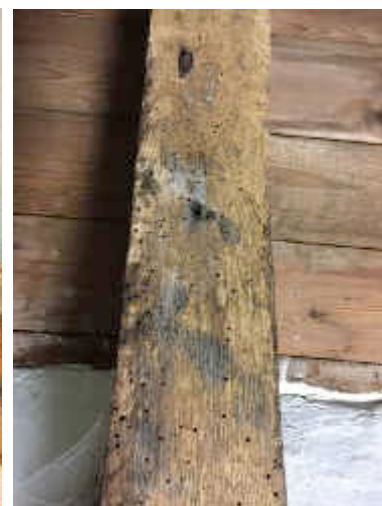
Figure 80 ~ Details of typical soiling and discolouration observed across the roof timbers.
