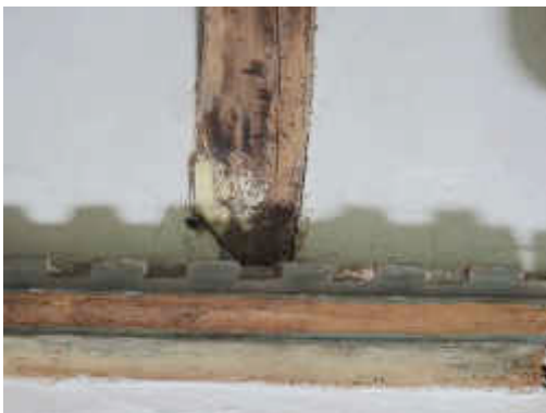
Figure 97 ~ The fine dentil carving of the wall plate in the nave have worn or been lost in areas and the upper section of some have been covered with a plain length of timber.
