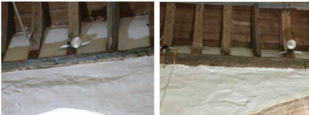
Figure 100 ~ Electrics and lighting have been fixed to timberwork above the wall plate line.
