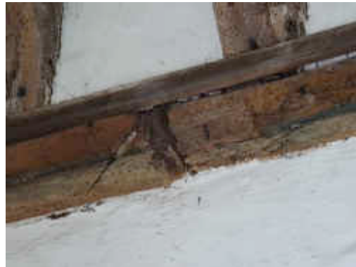
Figure 97 ~ The fine dentil carving of the wall plate in the nave have worn or been lost in areas and the upper section of some have been covered with a plain length of timber.
