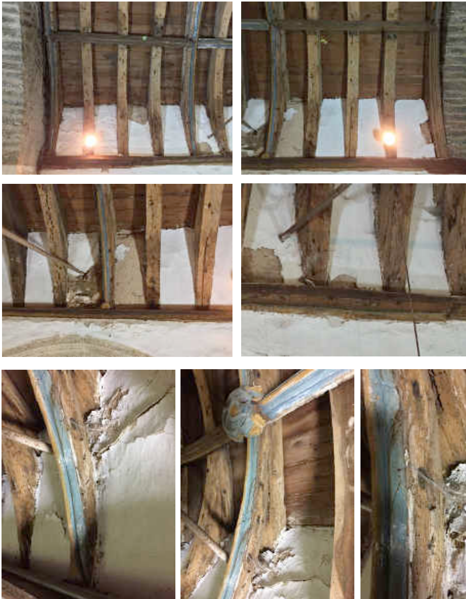
Figure 83 ~ Areas of detached and flaking plasterwork observed at the west end of the south
