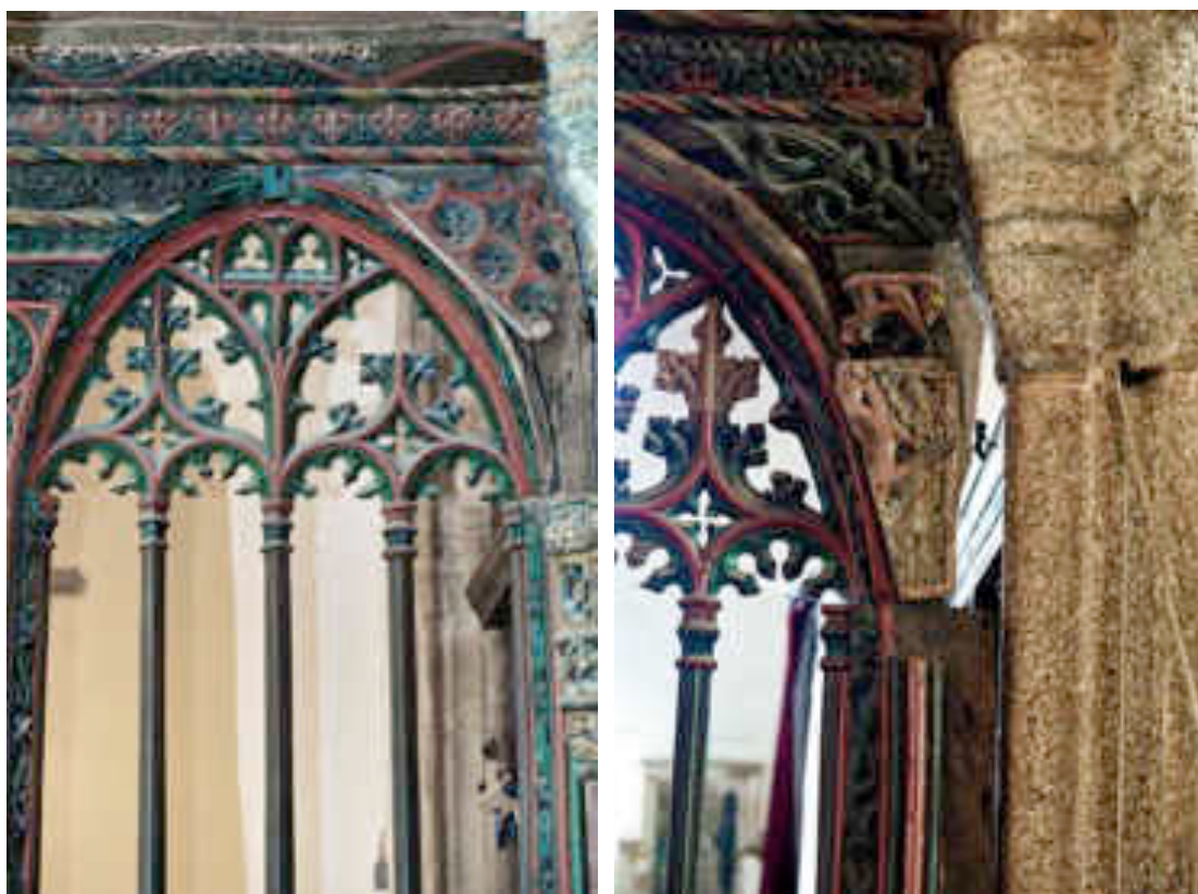
Figure 47 ~ Sections of carvings have been repositioned within the flattened spandrels (top left & right) and run of moulding are misaligned with inconsistent gaps (below left & right).
