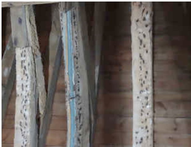
Figure 85 ~ Areas of ribs with larger number of nail holes. It has been presumed that this area was repaired with lath and plaster at some point. A leak in the roof may have caused the original panelling to fail.
