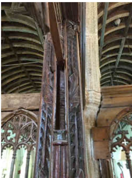
Figure 63 ~ Chiselled out channels in framework, indicating location of tracery sections now missing (left) and length of square section timber pieced in to offer support to vulnerable tracery (above).
