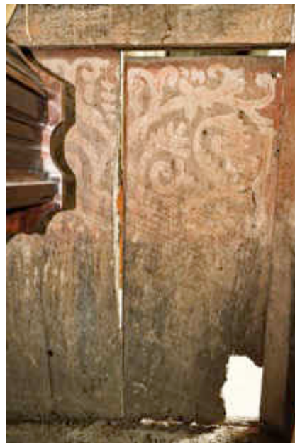
Figure 36 ~ Details showing various areas of losses and vulnerable sections observed across the rood screen.
