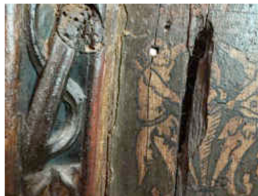
Figure 37 ~ Cracks and damaged sections noted on the painted dado panels on the south aisle screen.
