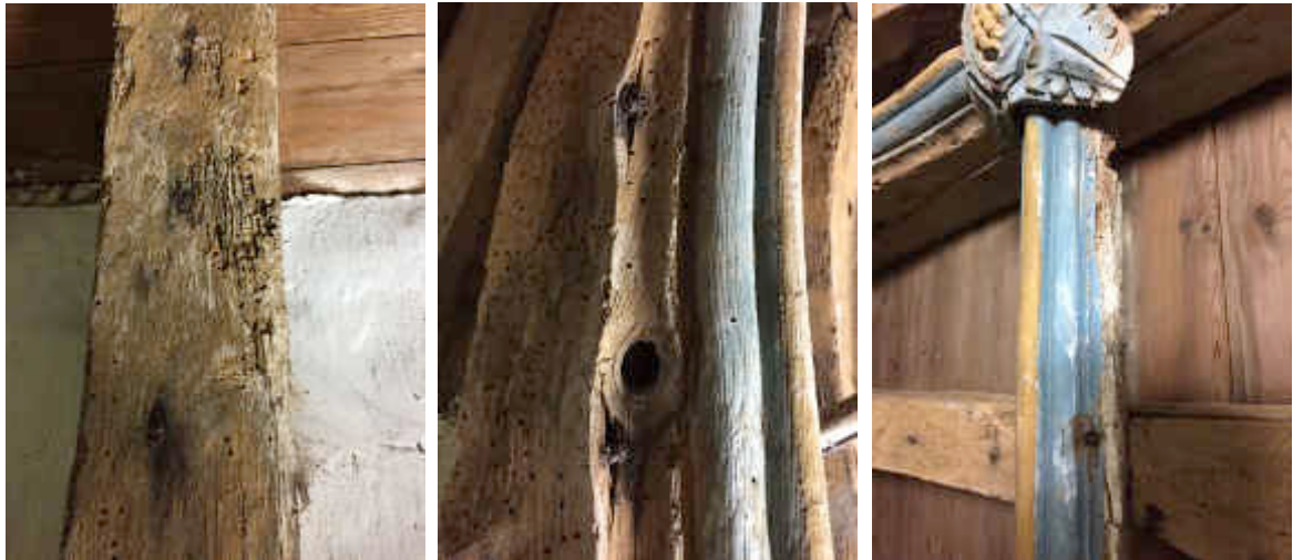
Figure 88 ~ Staining and splits to timberwork observed as a result of corroding ferrous fixings.
