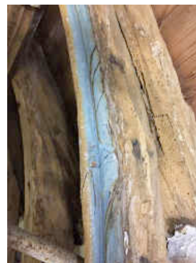
Figure 79 ~ Details showing staining from past leaks.
