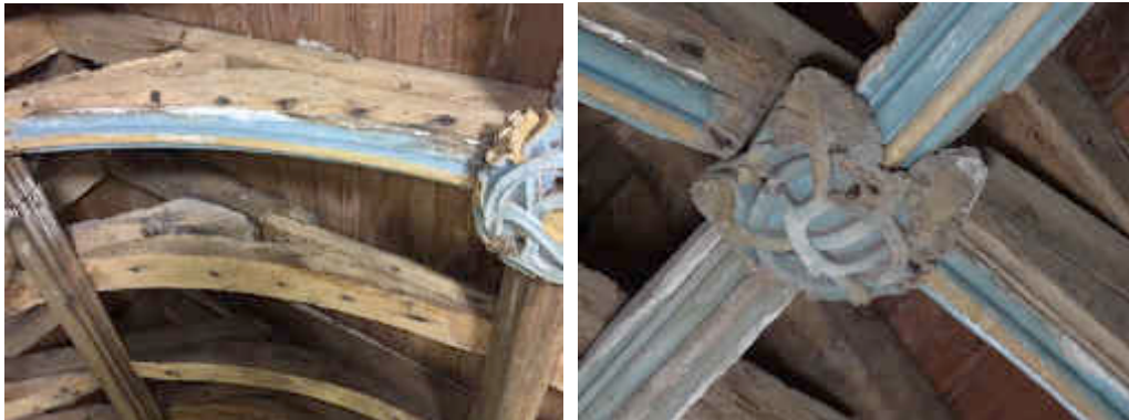
Figure 99 ~ Corroding ferrous fixings have stained adjacent timberwork.
