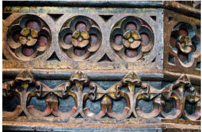
Figure 64 ~ Details showing the overall dulled appearance of the polychromy due to surface dirt and dust and discoloured varnish layers. The dirt layers have accumulated within later surface coatings.
