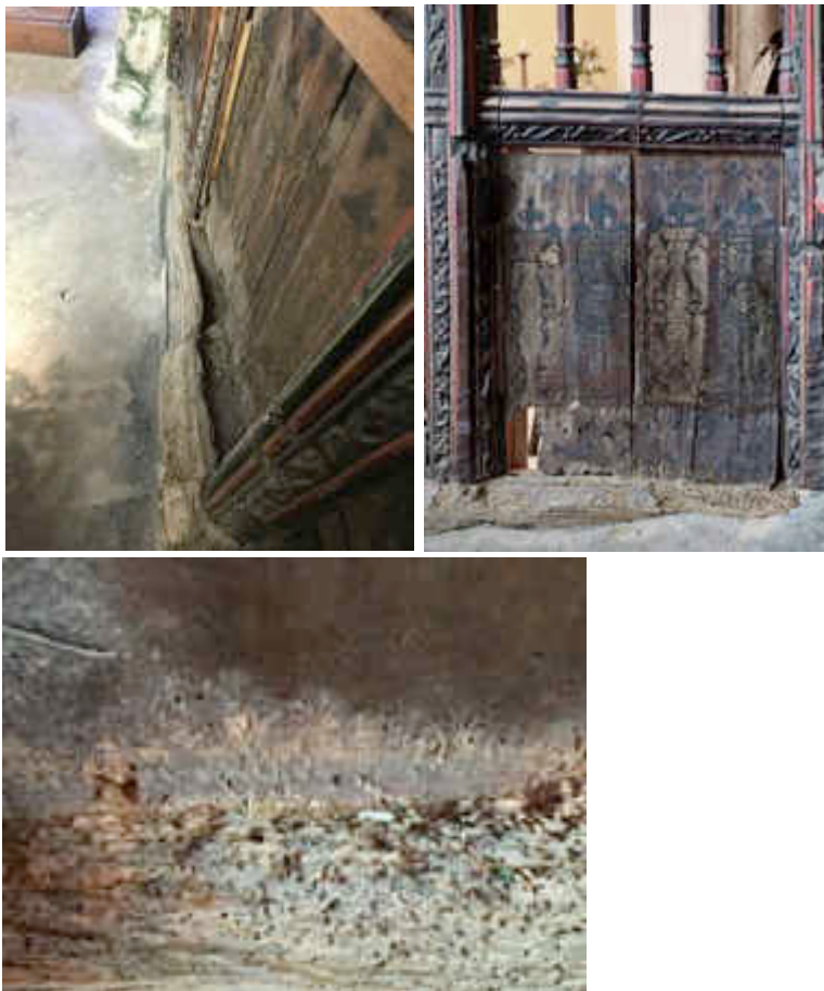
Figure 35 ~ Evidence of insect damage was observed across the timber screen.
