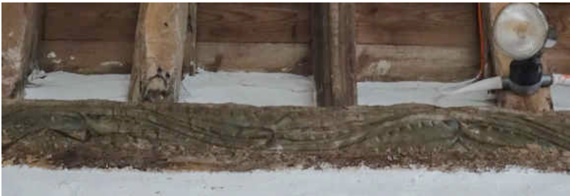
Figure 29 ~ Detail of more elaborate vine scroll wall plate design noted along south elevation of Lady Chapel.
