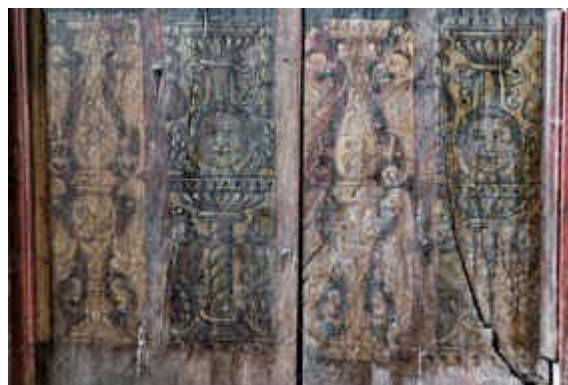
Figure 44 ~ The panels on the west elevation of the north aisle sections of the screen have been coated with a varnish. As noted elsewhere this coating has been thickly applied with dark drip runs observed.
