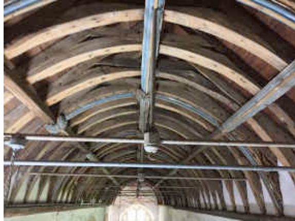
Figure 95 ~ Tie rods were introduced across all three areas of roof timbers during an earlier Victorian phase of repair.
