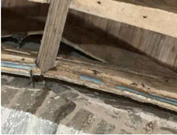
Figure 84 ~ losses to the timber structure in general and to the wall plate line (above right) were observed throughout the church.
