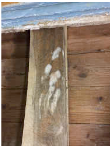
Figure 80 ~ Details of typical soiling and discolouration observed across the roof timbers.
