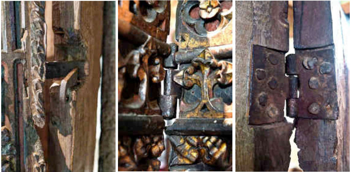
Figure 73 ~ Details of ferrous fixings on the pulpit showing signs of corrosion but relatively stable.
