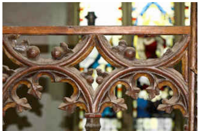
Figure 63 ~ Chiselled out channels in framework, indicating location of tracery sections now missing (left) and length of square section timber pieced in to offer support to vulnerable tracery (above).
