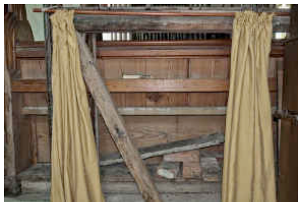
Figure 14 ~ North elevation of parclose screen between chancel and Lady Chapel to the north, showing upper section (right) with carved tracery and lower section (above) with missing timber panels.
