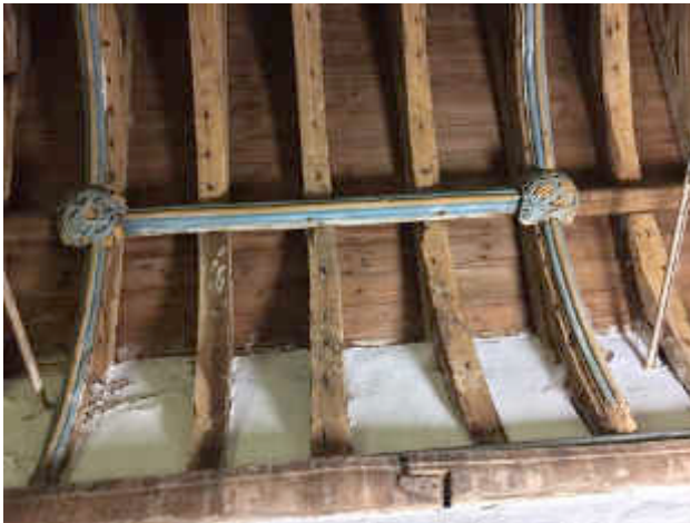
Figure 96 ~ Timber panelling lost from between the moulded purlins and ribs.
