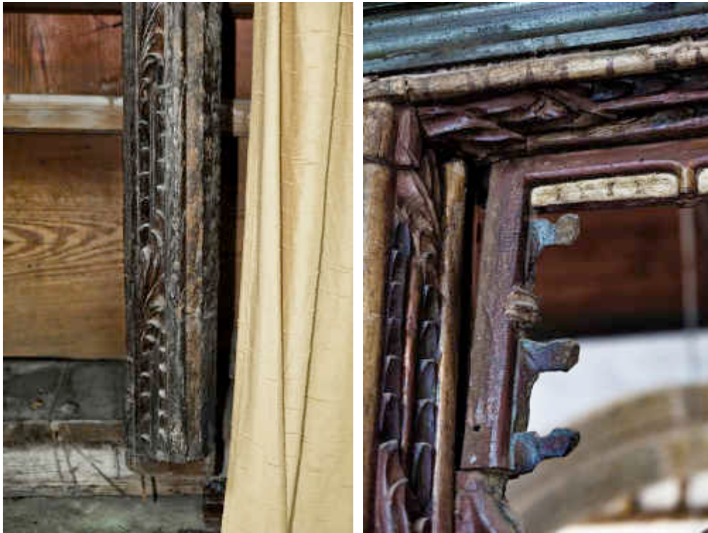
Figure 58 ~ Details showing missing support to the base of carved upright post on north screen (left) and dropped / misaligned section of tracery on north screen (right).
